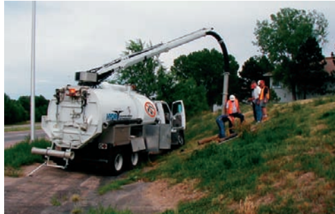
Water Shutoff Repair
