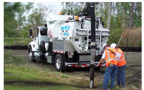
Day Lighting Buried Utilities
