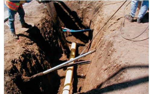
Multiple Utility Lines Safely Exposed
